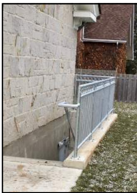
New fire safety exit from basement for staff
